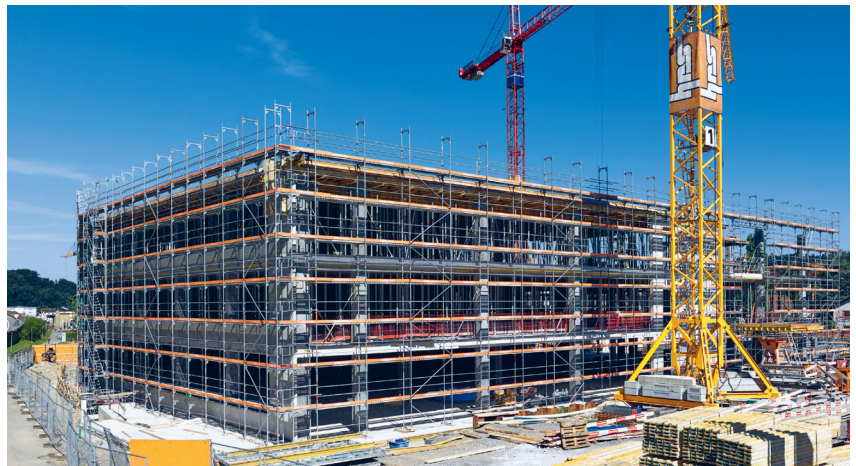
Facility expansion in Flamatt: ready for occupancy in late summer 2018
